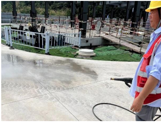
施工期洒水抑尘
