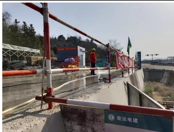
施工期洒水抑尘
