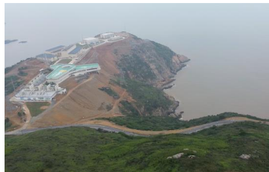
拟建站址东侧
